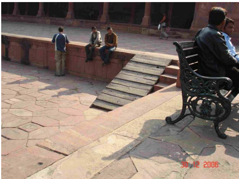
Picture 4: Another view of the 3 rd ramp from the entrance – the spoil sport
